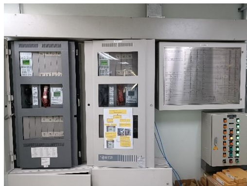
fire alarm control Panel
